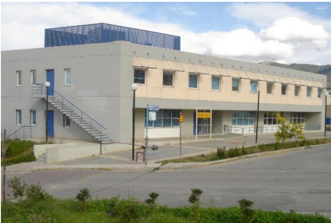
Building of the Laboratory for Structural Analysis and Antiseismic Research
