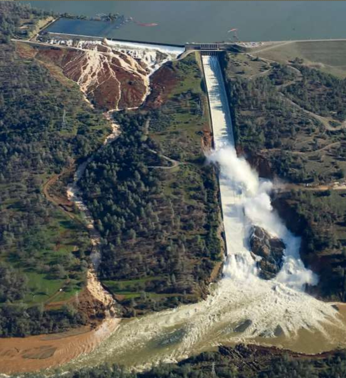
Oroville Dam, spillway damage, Feb 2017
