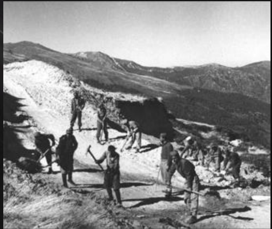
Greek Army engineers repair a road.
