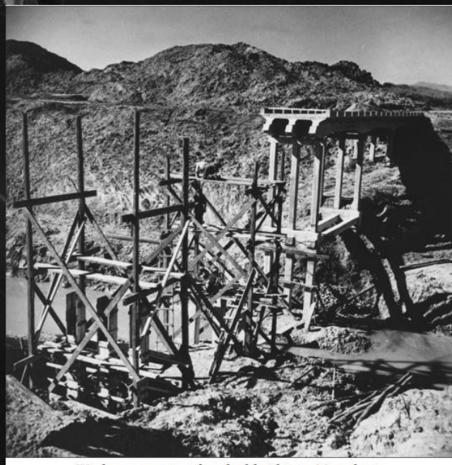
Workmen repair a bombed bridge in Macedonia.
