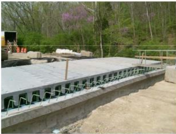
Industry's first integrally molded FRP bridge
