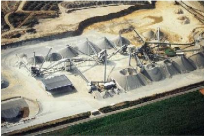
Aerial view of a typical aggregate production plant.
