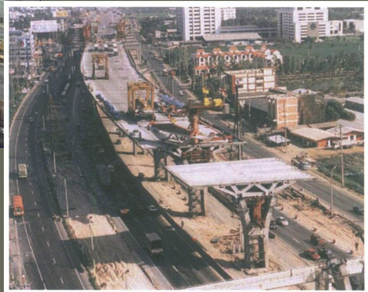
Fig. 18. Overview of progress in erection of bridge superstructure.
